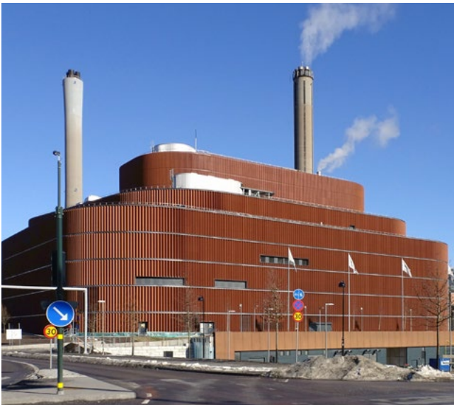
Fortum's new bio-fuelled CHP plant in Hjorthagen, Stockholm. Photo by Holger.Ellgaard / CC BY-SA 4.0
